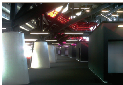
Figure 6. Podium concourse under completed upper tier showing vomitory stairs with coloured glass barriers and toilet pods
