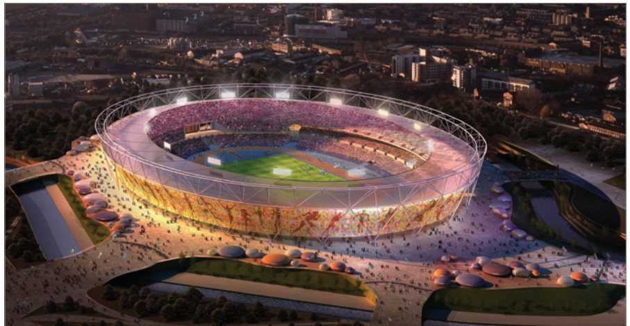
Figure 1. Final concept submitted for planning approval, showing the sporting arena on the constrained island site with spectator facilities located in pods outside the main structure
