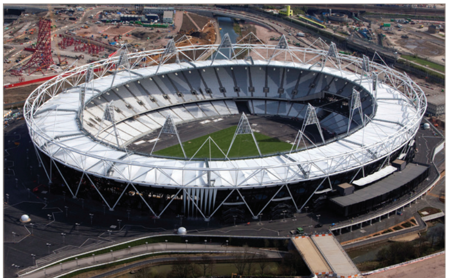
Figure 9. The stadium was completed on schedule and within budget in March 2011 – note prototype 'wrap' panels in foreground, west stand pavilion to lower right and initial external pods
