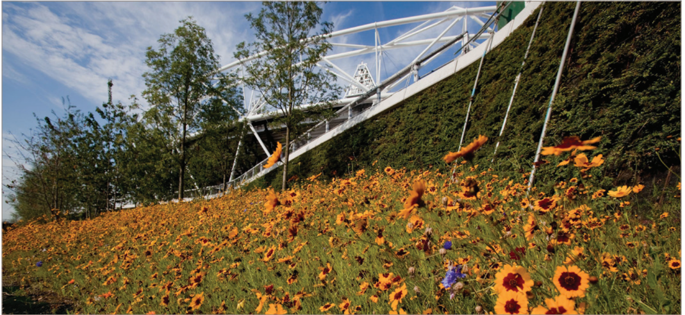
Figure 11. Strengthened earth embankments provide soft green edges around the stadium
